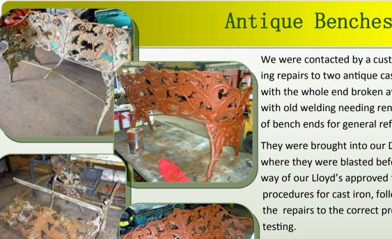
We were contacted by a customer regarding welding repairs to two antique cast iron benches – one with the whole end broken away, and the other with old welding needing renewing—and also a pair of bench ends for general refurbishment.
