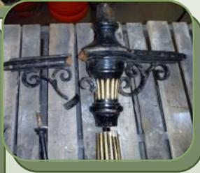
One of the cast iron columns was very badly damaged, and needed our expertise in carefully piecing it back together, using our Lloyds approved fusion welding procedure. This was followed by grinding of all welds to match existing shape, then blasting and finally given a good coating of red oxide primer before returning to Sugg & Co for their final restorations to the gas lamp, and shipping back out to Hong Kong for reinstallation.
