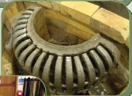
A rare feature of this water crane was the fire basket, which would prevent water from freezing in extreme cold temperatures, and also stop the cast iron from cracking...many of the original fire bars were missing, so a pattern was made from a good part of the casting and sent away to our trusted foundry to have the basket recast. Once cast, it was welded in and ground to shape before shot blasting and painting with red oxide primer and undercoat.
